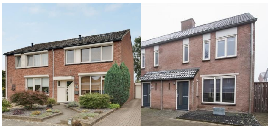
Figure 2: Examples of semi-detached dwellings built between 1965 and 1974.
