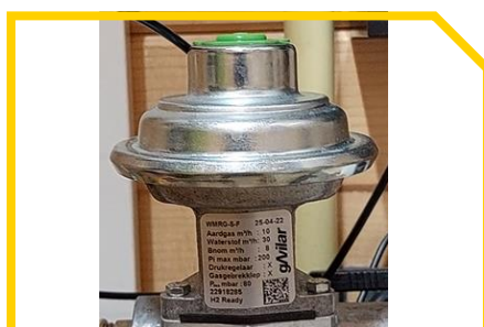
Gas pressure regulator green cap
