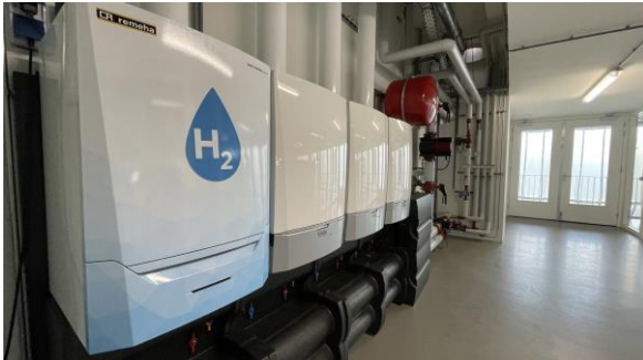
Demonstration project with 45 kW 100% hydrogen boiler for utility building 2023
