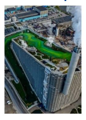
The CopenHill in Copenhagen is a new breed of waste-to-energy plant topped with an artificial ski slope and world's highest climbing wall of 85 meters. Beneath the slopes, furnaces and turbines convert 440,000 tons of waste annually into enough energy to deliver electricity and district heating for 150,000 homes.
