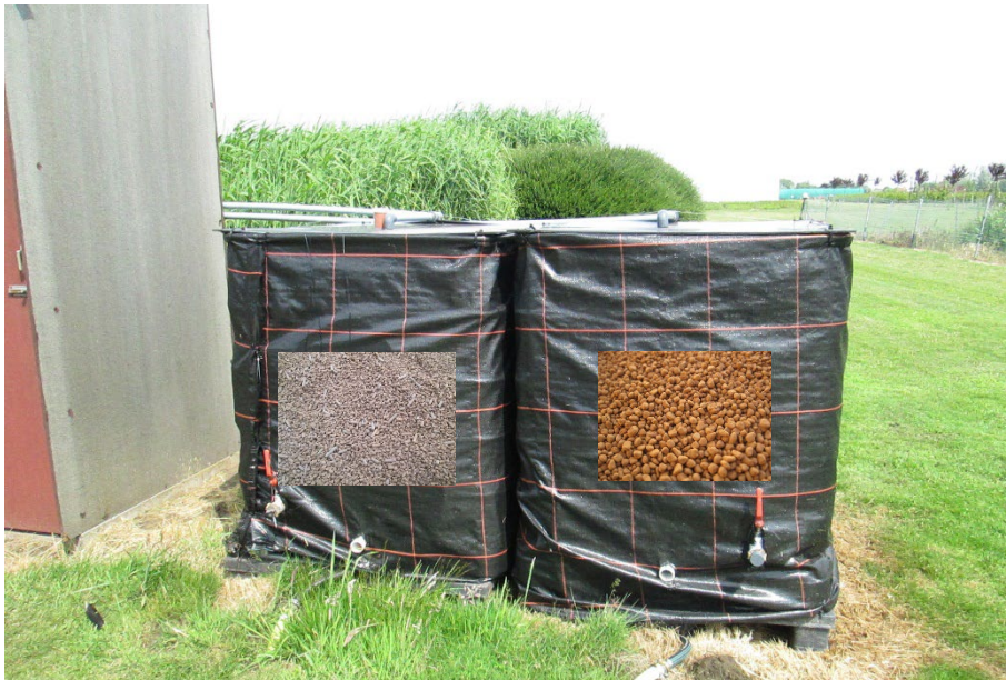
Photo 2 Two P filters at PCS (in parallel)
