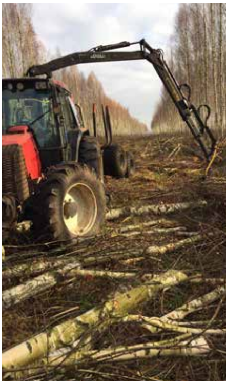
Clearing of woody vegetation at Amalva peatland. Photographer: Z.Sinkevicius for LIFE Peat Restore
