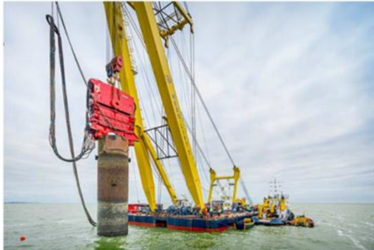
Figure 20 Vibratory extraction of monopile (decommissioning of Lely wind farm) [16]
