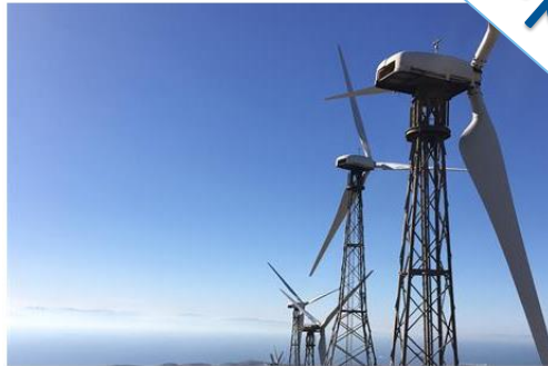
The 30MW El Cabrito wind farm currently comprises 90 330kW turbines (pic: Nordex)
