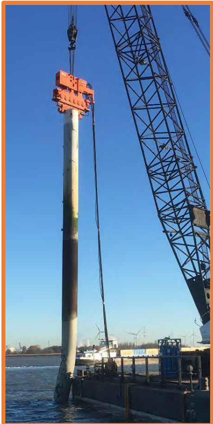
Removal of damaged piles
