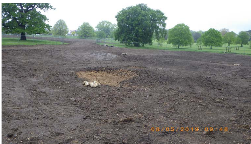
Final shaping of wetland cells with topsoil including formation of bund, deep pools and islands (early May 2019)
